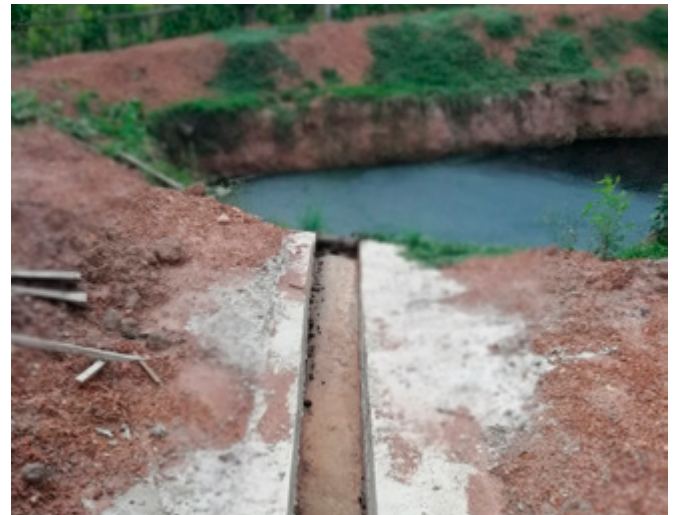
Dao's new pig shed was designed with help from the District Agriculture and Forestry Office. The sloping concrete floor makes it easier to keep the pens clean, and slurry is channelled into a pond where it is stored until the dry season to be spread on nearby rice fields.
